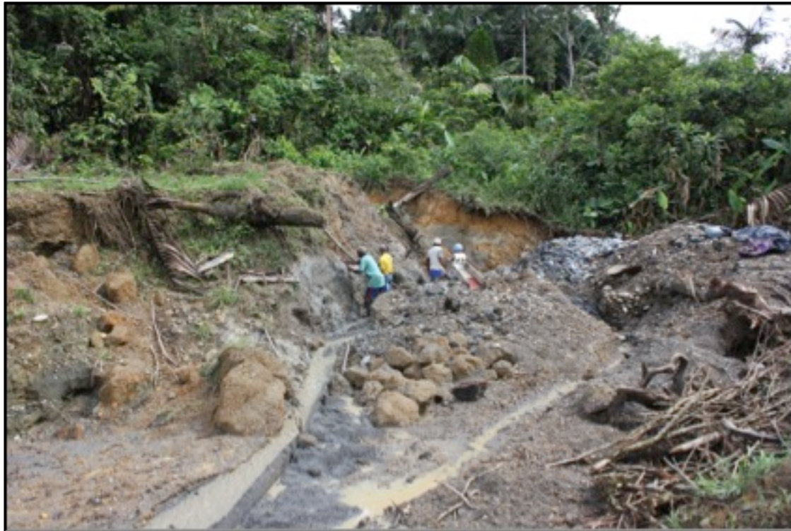
Picture 5. Removing soil
